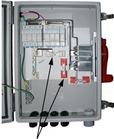
Remove Positive and Negative blocks and set aside. This is to provide access for the next steps.
