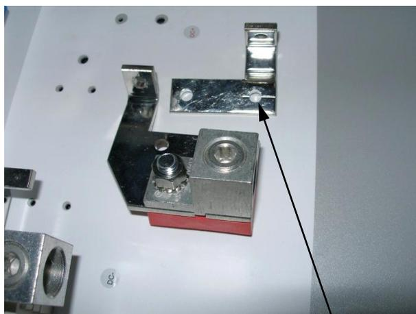
Remove two bolts holding small busbar.
