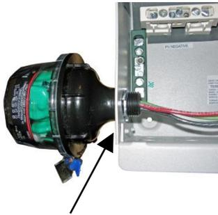
MNSPD Shown installed in left side knockout.
