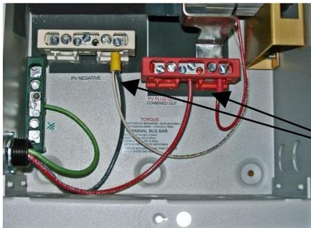
**Step 7a:** Strip the other end of the red and white wire about  $\frac{1}{4}$ ". Install the red wire into the red terminal block. Put the white wire along with the black wire from the MNSPD into the ferrule and crimp. If no MNSPD is installed the white wire may go directly into the white terminal block.
