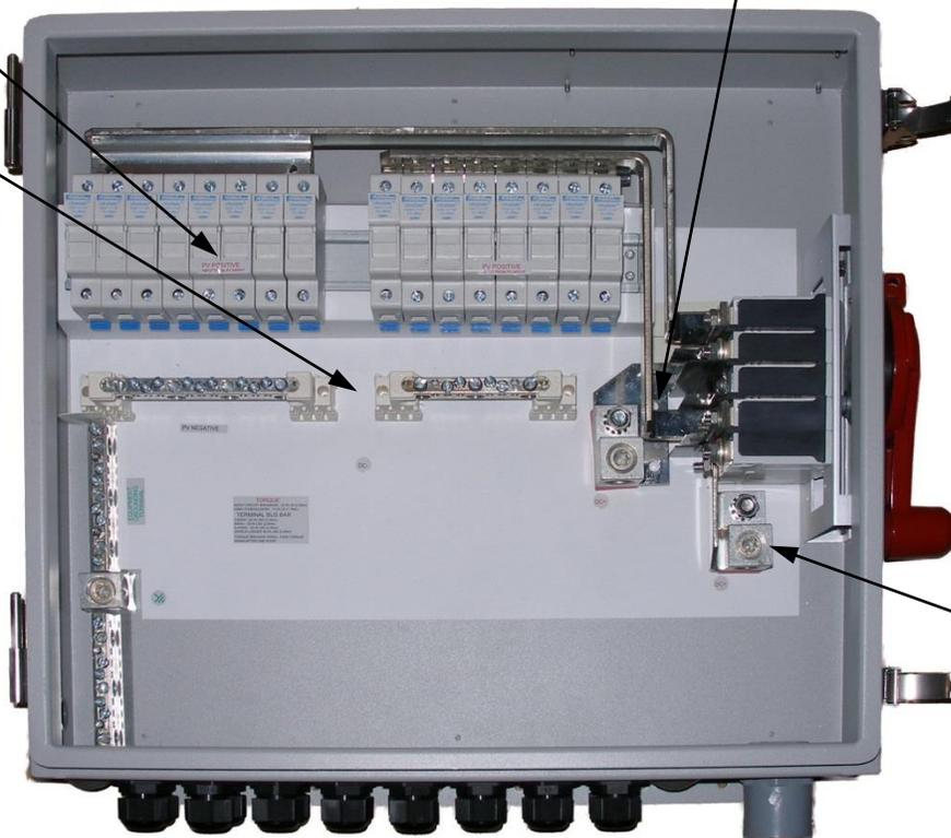
Second PV Positive output lug installed
