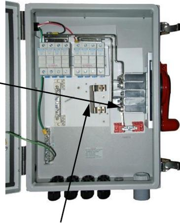
Remove Positive jumper busbar from switch, set aside, it is not used in this configuration. Replace nut on lowest position only
